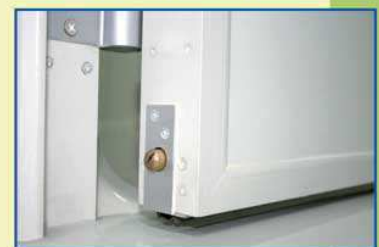
Door's drop-down bottom seal to prevent air transfer
