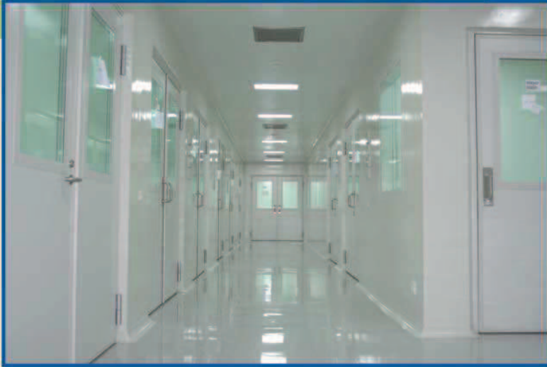
A Clean Room corridor in a pharmaceutical company
