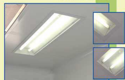
Inbow lamps specially designed for clean room
