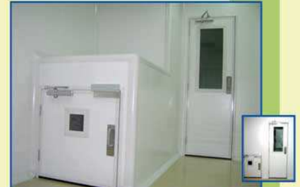
Pass Box from inside a Clean Room. Inset: from outside
